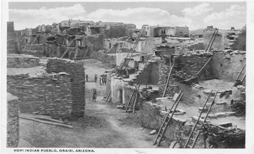
Figure 3: The Hopi Pueblo of Oraibi, perched on the Third Mesa of Arizona, from a postcard, ca. 1920. Upper stories of houses were reached by ladders or stairs on the outside
